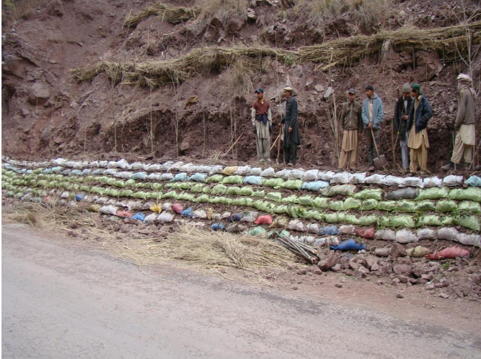
Land Stabilization under One UN DRM Joint Programme (NDMA/UNDP-Pakistan)
